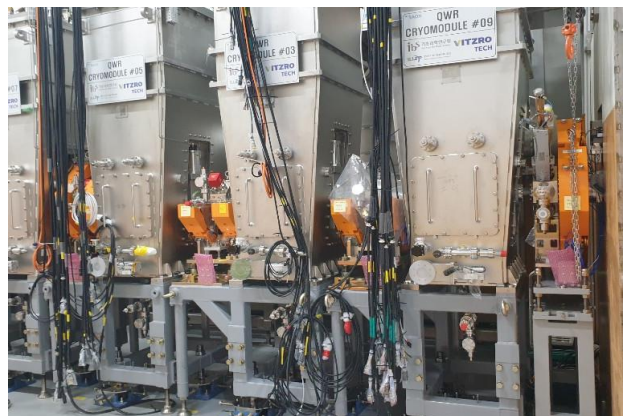
Figure 3. The first few cryo-modules in which a superconducting cavity is assembled, are connected with warm section components during installation
