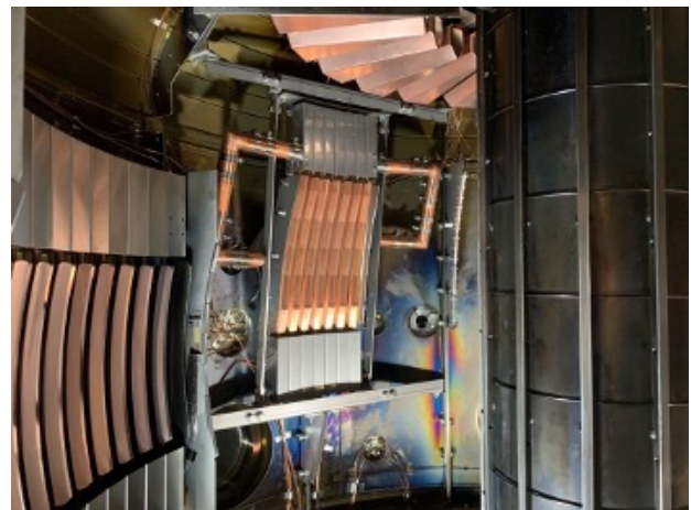
Figure 1. The newly installed off-midplane launcher (center) with the previously installed midplane launcher (left) and top launcher (top).
